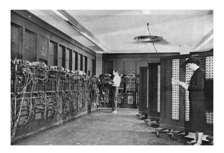
This is the first electronic general-purpose computer, the ENIAC, which was built at the University of Pennsylvania between 1941 and 1946. It was used extensively for Edward Teller's early work on hydrogen bombs. The size of a couple of rooms, it had thousands of components and millions of hand-soldered connections.
